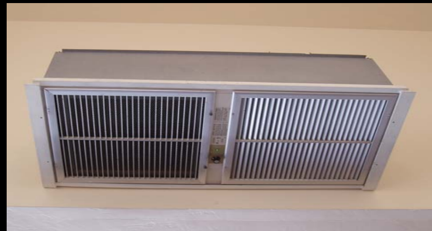
ESP mounted on ceiling
